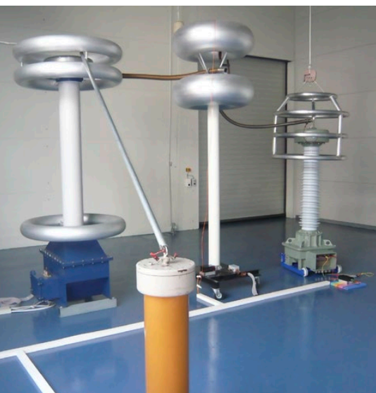
300 kV high-voltage laboratory PFIFFNER Instrument Transformers Ltd. / Switzerland
